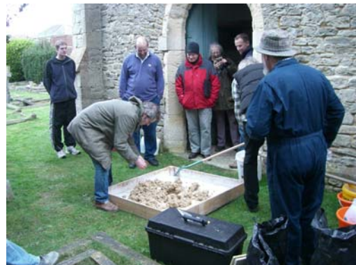
Above: Ray Moseley and Kevin Stubbs from Bursledon Brickworks demonstrating the use of lime mortar in building repairs
