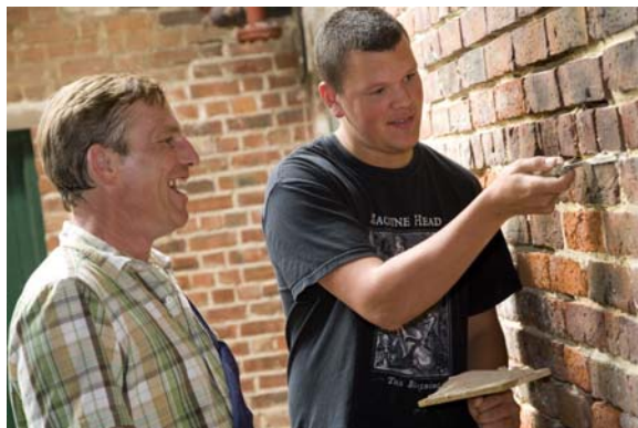
Above: Ray Moseley and Kevin Stubbs from Bursledon Brickworks demonstrating the use of lime mortar in building repairs
