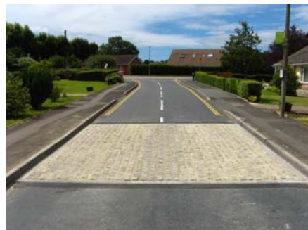
Works undertaken 2006/07 – Gateway treatment and traffic calming, Hinton Road. Carisbrooke
