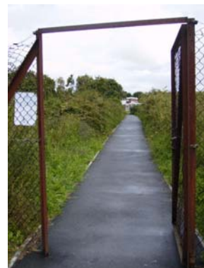
Works undertaken 2006/07 – New footway linking St Thomas’ School, Carisbrooke to existing right of way
