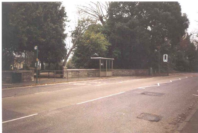
Figure 2.8 - Poor Quality Bus Infrastructure
