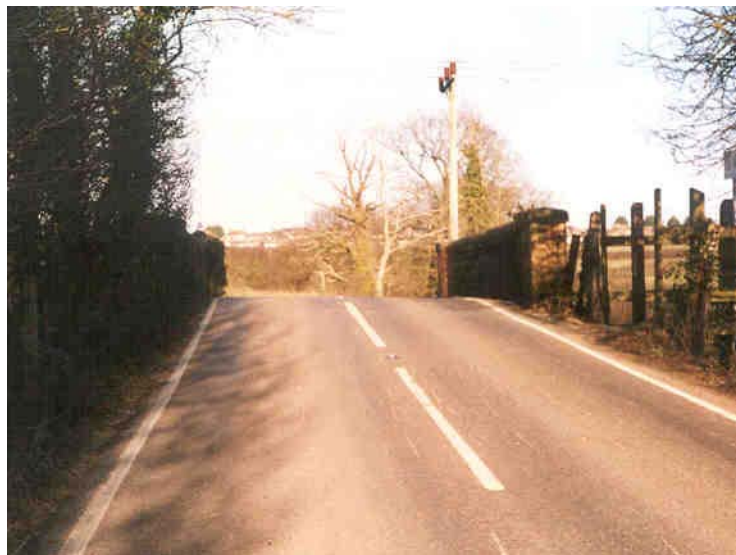
Figure 7.4 – Railway Bridge on Smallbrook Lane
